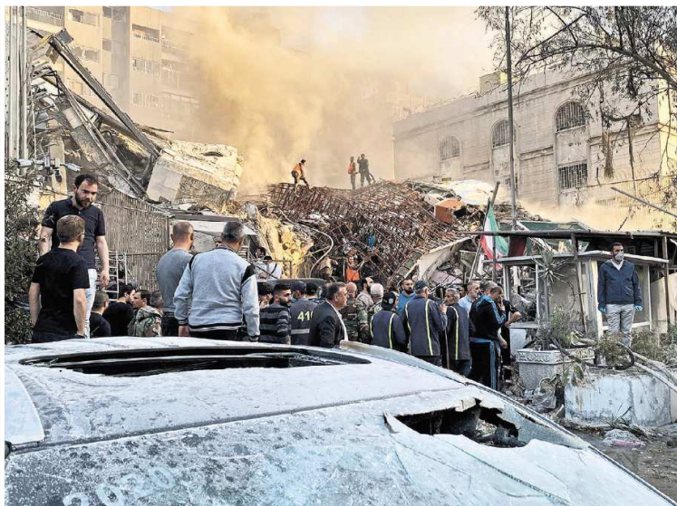
The aftermath of an Israeli attack on Monday on a building that Iran said was part of its embassy complex in Damascus, Syria.
