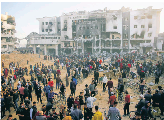
STRICKEN: Palestinians inspect damage outside Gaza's Al-Shifa Hospital after the Israeli military withdrew on Monday following two weeks of heavy fighting to root out Hamas forces there, leaving much of the hospital destroyed. A5
